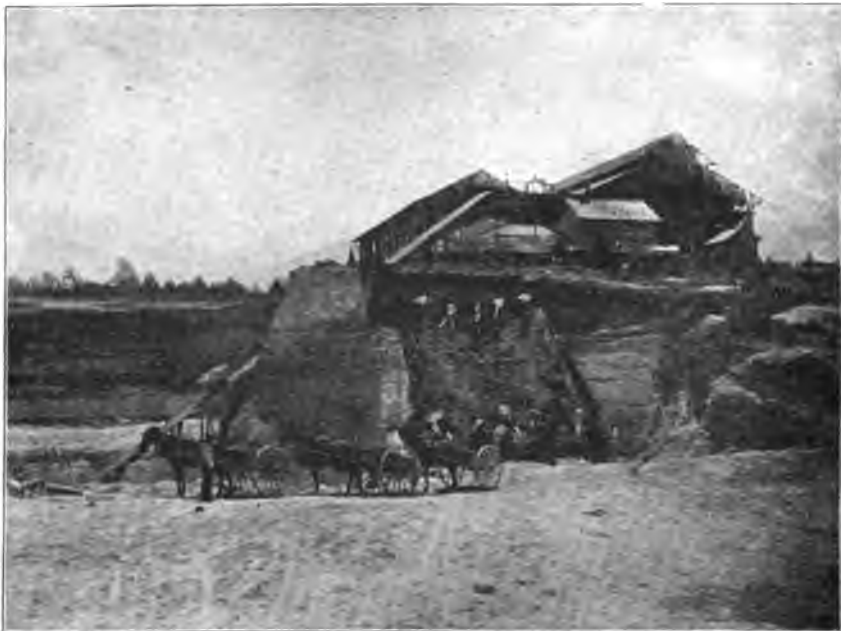
SEDIMENTARY KAOLIN MINE—REMOVING THE OVERBURDEN.
